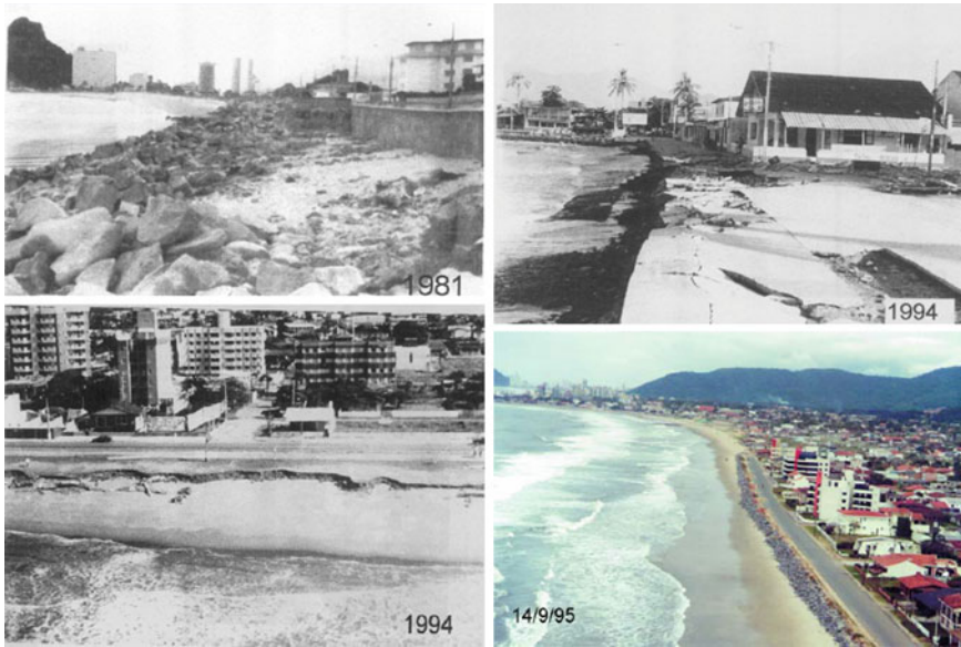
Fig. 24.8 Photos of the shore in 1981, 1994, and 1995. Walls of concrete were applied as protective tools against the encroaching ocean. Source Angulo et al. (2000)
