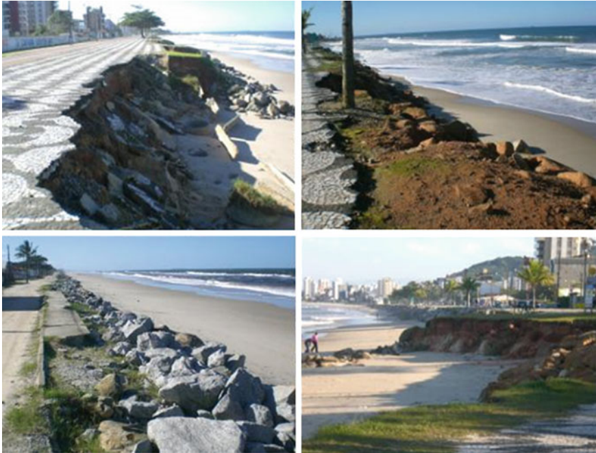
Fig. 24.3 Impacts of shoreline erosion in Matinhos District in the coast of Paraná State, Brazil in 2007. Source Goncalves (2010)
