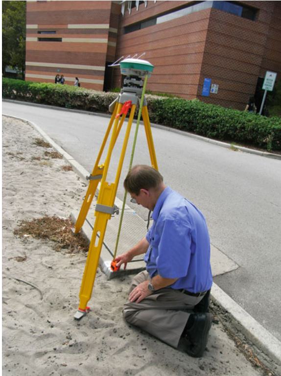
Fig. 6.6 Setting up an antenna and measuring its height at Station John Walker (JW) at Curtin University, Australia
