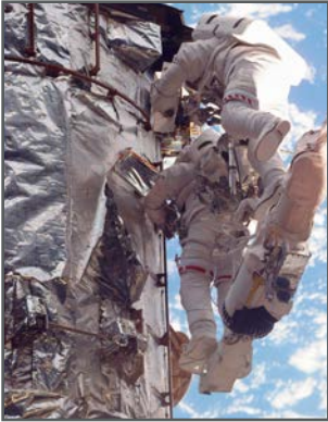
Large radiation-induced cracks in the outer layer of multilayer insulation after 6.8 years of space exposure (Townsend et al., 1999).
