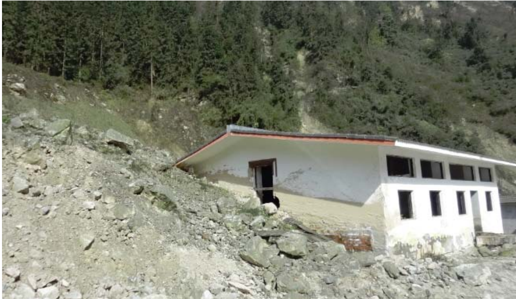
Figure 5.2 Landside damage in Sichuan, China, 2010
